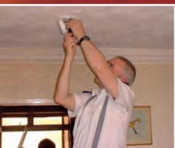
A firefighter replaces a smoke alarm that was damaged while alerting occupiers to a fire.
